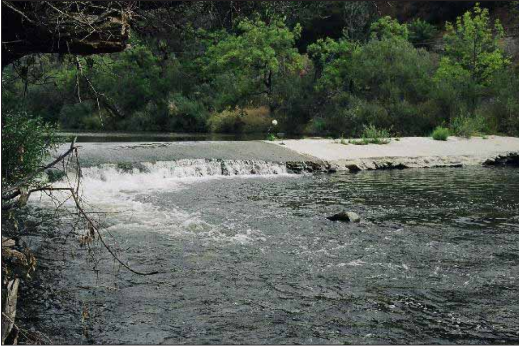
Figure 1 - The Alameda Creek near Niles flow measurement weir during summer low flow.
