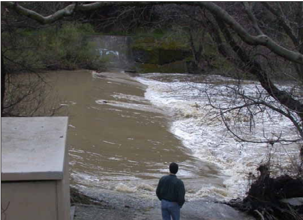
Figure 5 – The Alameda Creek near Niles flow measurement weir on 2/27/2006, 10:56 am at approximately 680 cfs.
